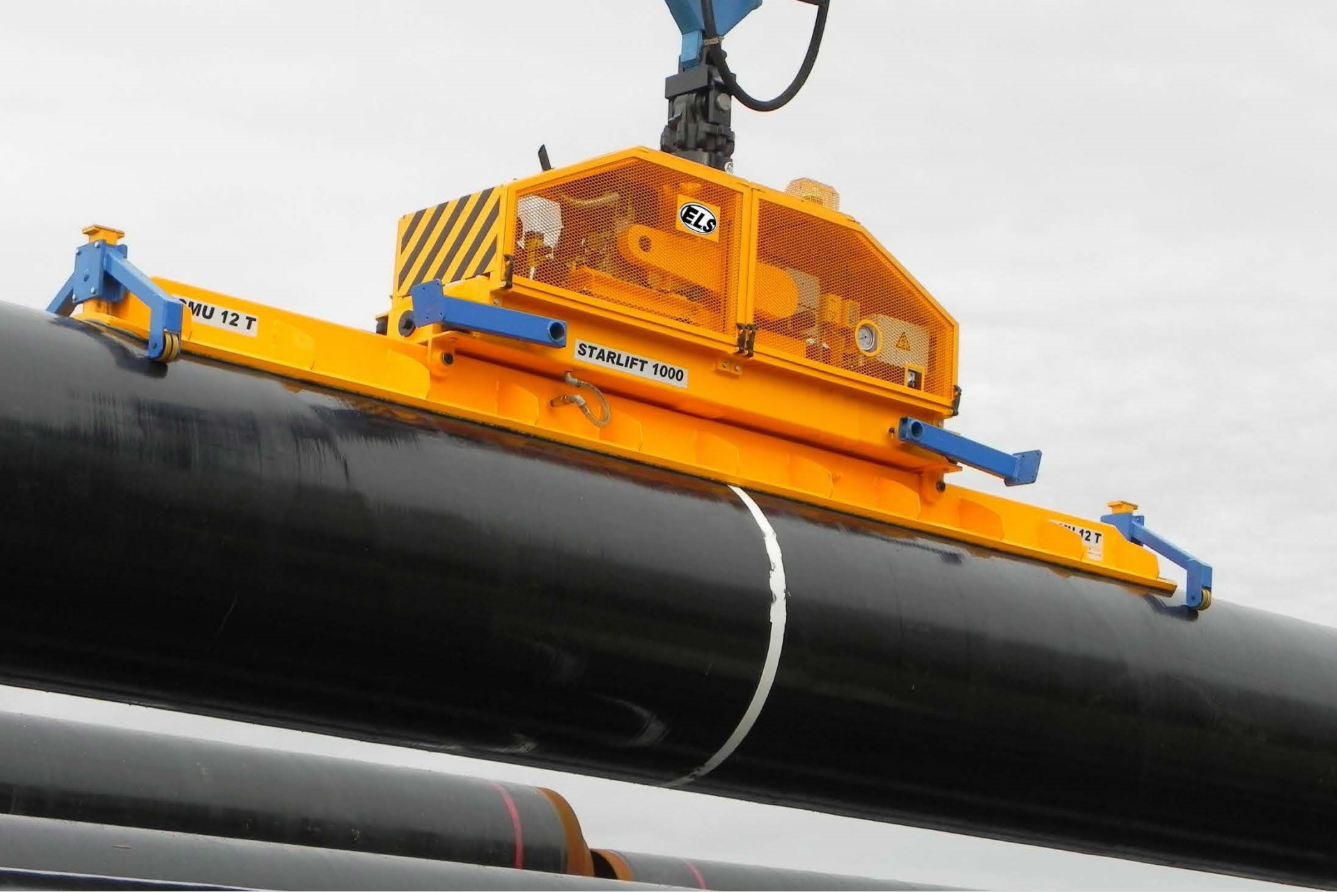
Pipe stocking 8m long & 48 inches & 5T
