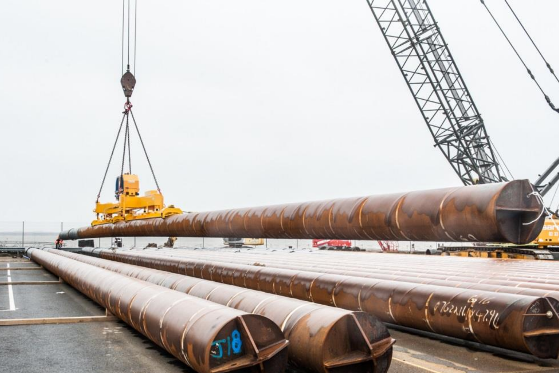
Oil pipeline 50m long 36 inches & 12 T
