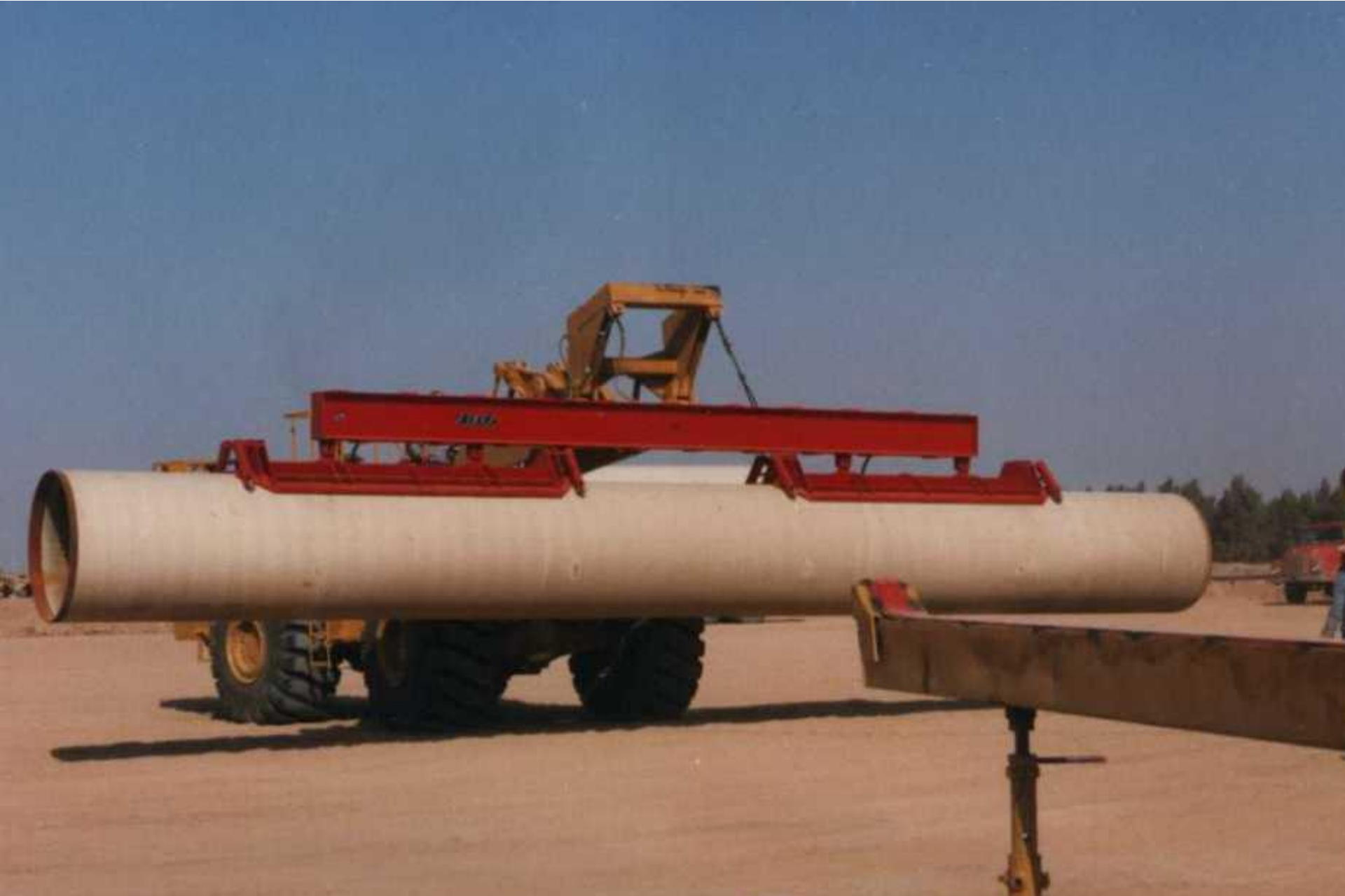
Water pipe 10m long 58 inches & 8T
