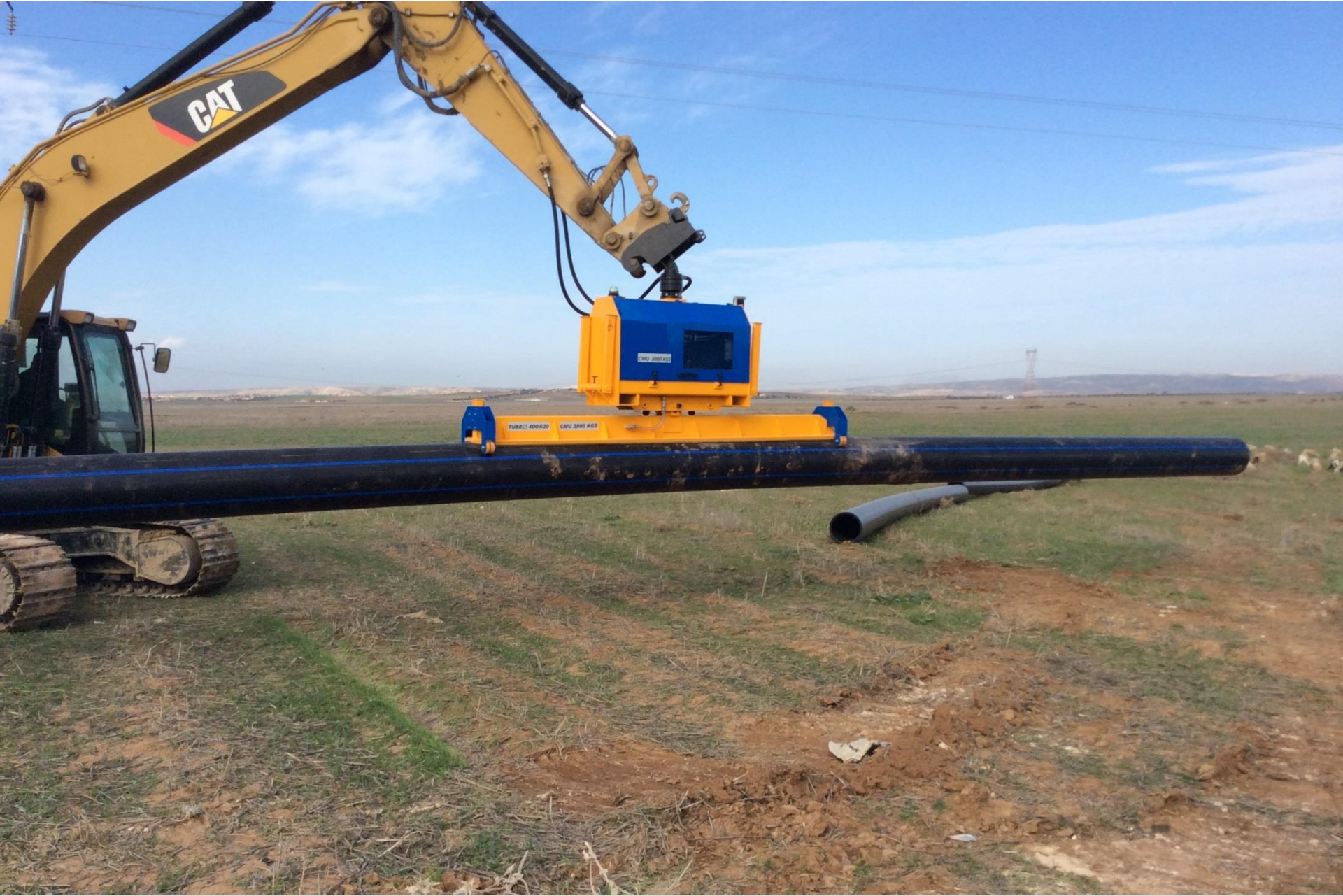
Water pipes 12m long & 12 inches & 800 kg
