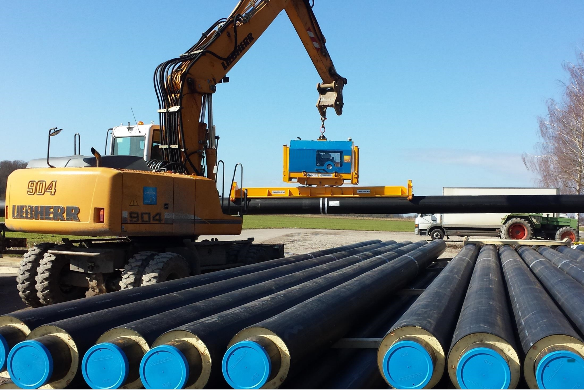
Hot water pipes installation 7m long & 12 inches & 2T
